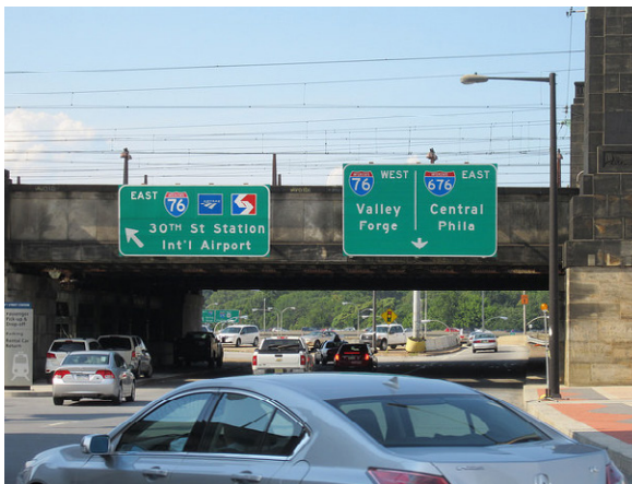
FOUR-LANE MERGE INTO A SINGLE-LANE ENTRANCE TO I-76/676 Credit: Parsons Brinckerhoff
