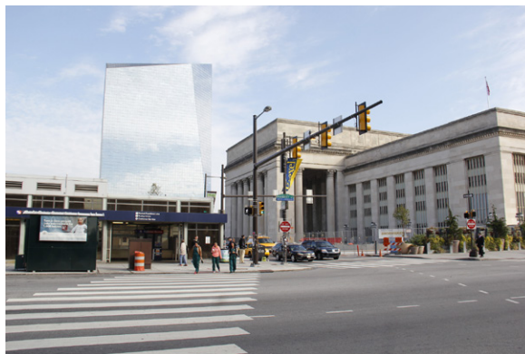
SEPTA SUBWAY AND TROLLEY STATION HEAD HOUSE Credit: Parsons Brinckerhoff
